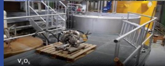
MELTSHOP - ZANESVILLE, OHIO
