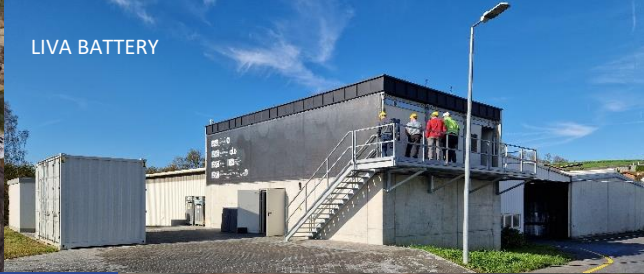
LITHIUM HYDROXIDE - BITTERFELD, GERMANY
